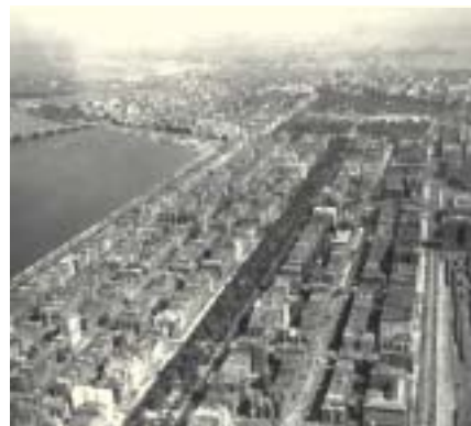
The Turnpike's Boston Extension, built along a railroad corridor, was completed in the 1960s.
