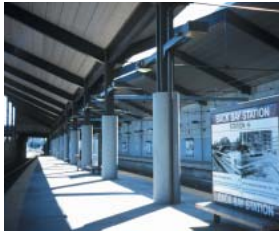
Commuter rail shuttles between Yawkey, Back Bay/South End and South Stations represent one of a series of significant public transportation investments.
