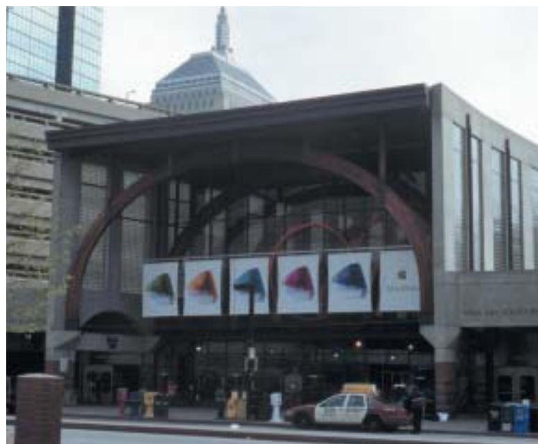
Back Bay/South End Station demonstrates how public transportation can enhance urban design quality.
