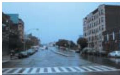
Existing conditions, Beacon Street.
