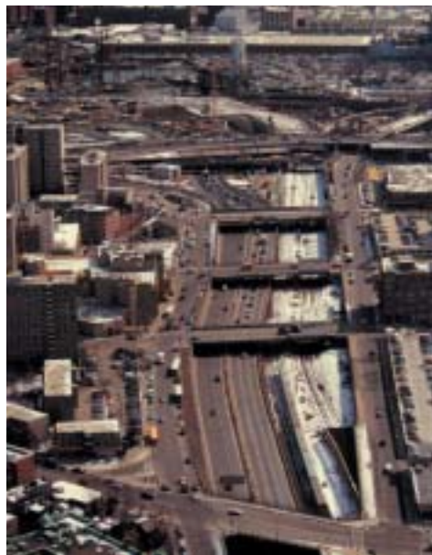
Air rights development would encourage much greater pedestrian activity along the cross streets—Washington Street, Shawmut Avenue, and Harrison Avenue.
