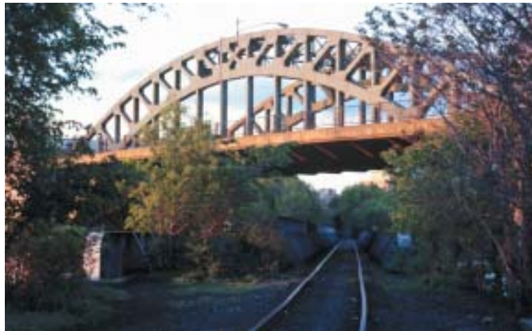
A path across Parcel 1 could connect pedestrians to both sides of the Charles River via the rail bridge.
