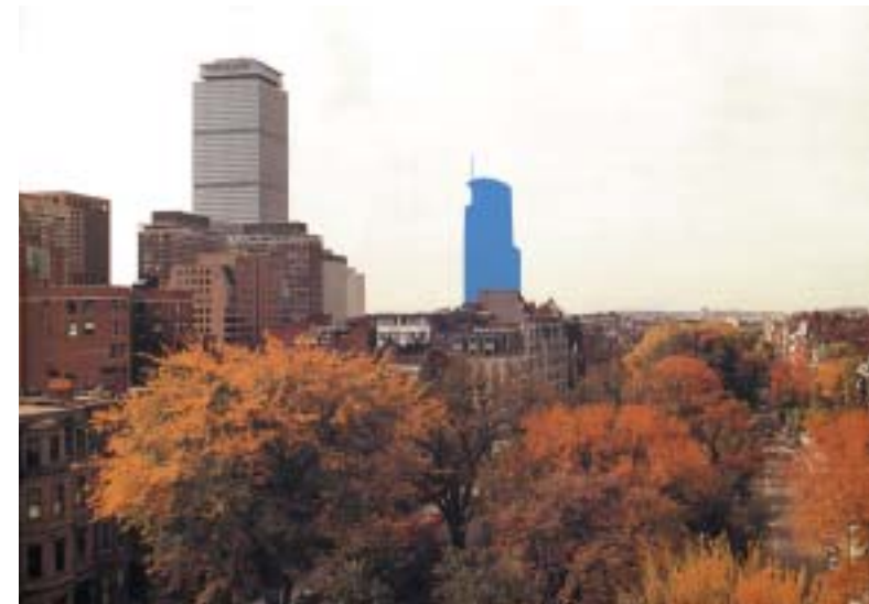
A taller building stands alone on Parcel 12 (above). A taller building on Parcel 15 (below) joins the collection of taller buildings that already mark the commercial Back Bay district.
